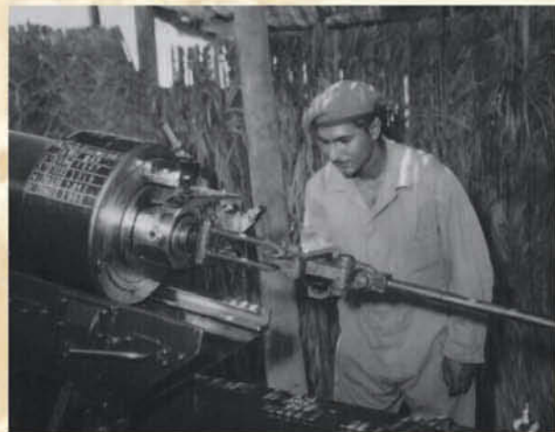
Right: EME Fitter at Bait Al Falaj checking the recoil system on a 5.5 Gun
